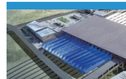
Intelligent Monitoring Solution for Shelters in High-speed Railway Stations
